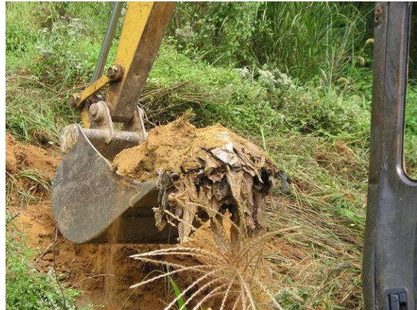
TP-136, Located Along Southern Landfill Property Boundary (Adjacent to WSSC Property)
