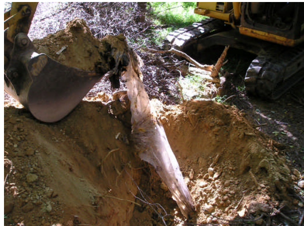
TP-8A, Located on M-NCPPC Property (Along N.E. Landfill Property Boundary)
