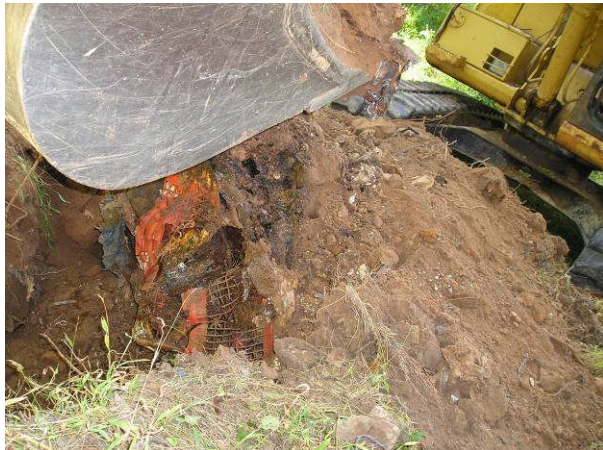
TP-5A, Located on M-NCPPC Property (Along N.E. Landfill Property Boundary)
