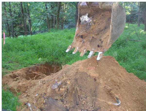
TP-48, Located Along N.E. Landfill Property Boundary
