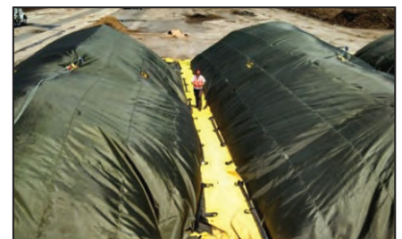
Example of covered aerated static pile composting using an engineered covering.
