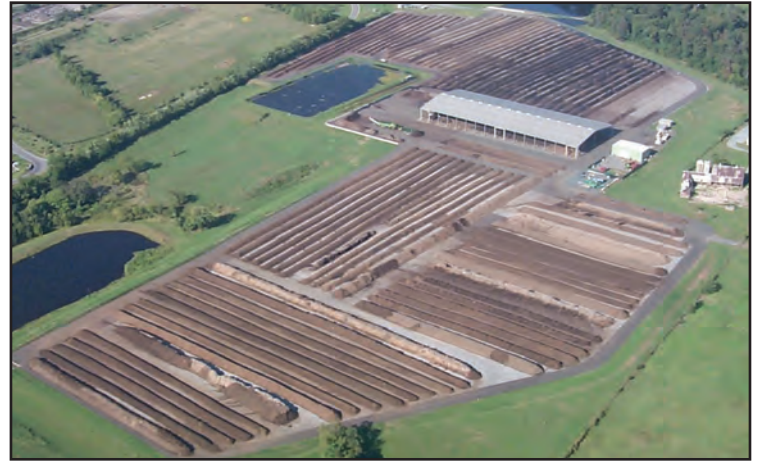
Aerial photo of the Montgomery County Composting Facility.
