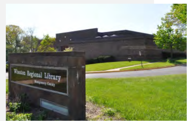
Wheaton Library built in 1962 , remodeled in 1985, removed "Regional" from original name
