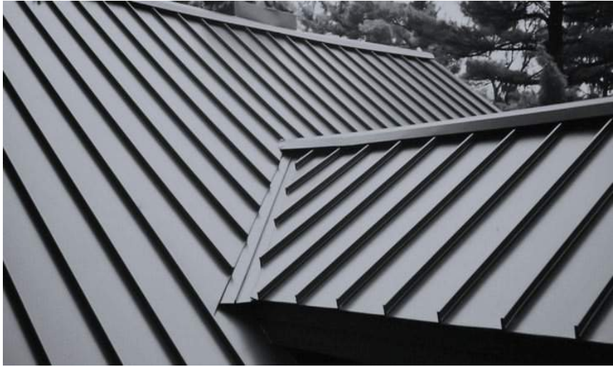
Standing Seam Metal Roof
