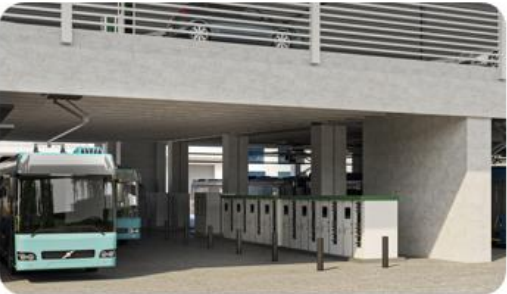
3. (10) 180 kW, (1) 360 kW BEB Chargers (5) 15 kW EV Chargers
