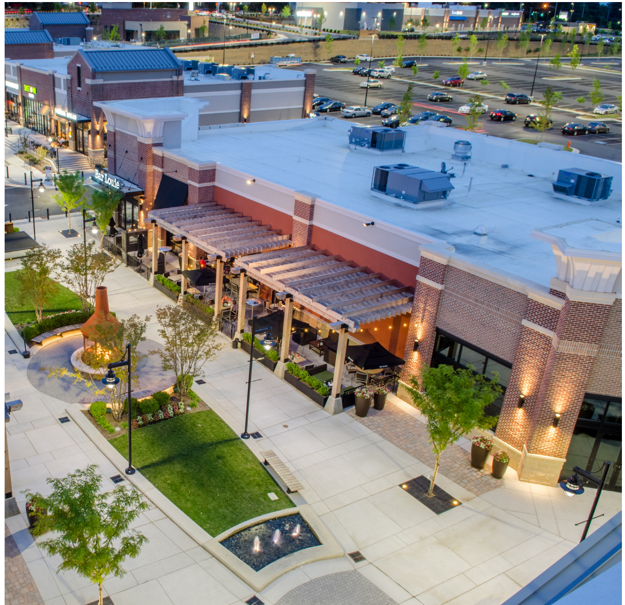
Mechanical equipment on the roof is set back an appropriate distance behind a raised parapet wall around the building's perimeter, so it is not visible from the street and adjacent parking lots
