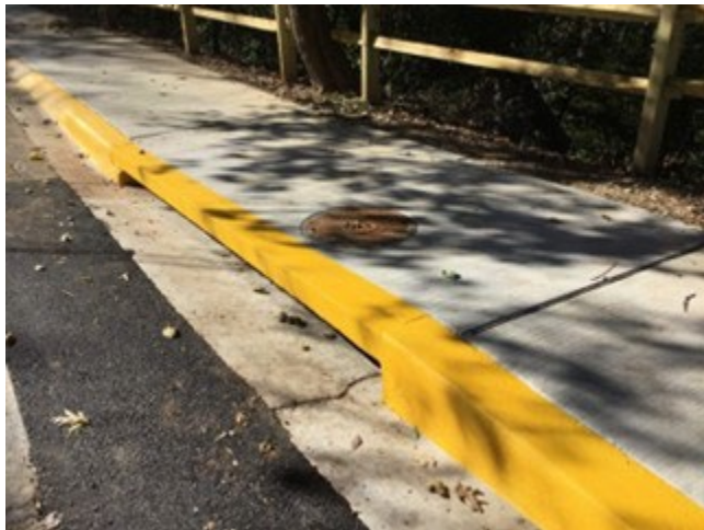
South Village Project Improvements Before
