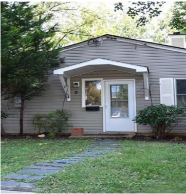
One of the original homes in Cabin John Gardens, a housing cooperative created in 1956 and probably Montgomery County's first common ownership community.
