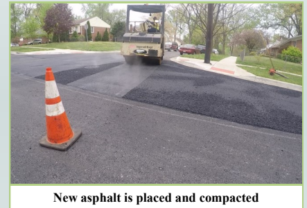
New asphalt is placed and compacted
