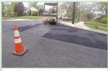
New asphalt is placed and compacted
