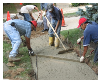
Concrete is smoothed and finished
