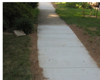
Completed sidewalk repair
