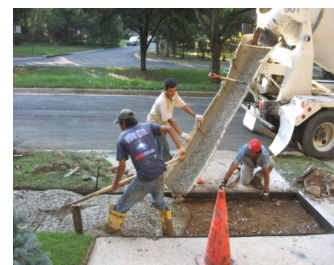
New concrete is poured into forms
