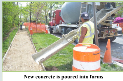
New concrete is poured into forms
