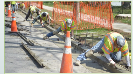
Concrete is smoothed and finished
