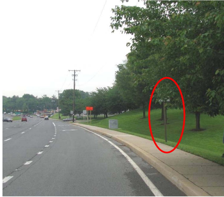
Tree canopy obstructs driver visibility of speed limit sign (circled) on southbound Connecticut Avenue.
