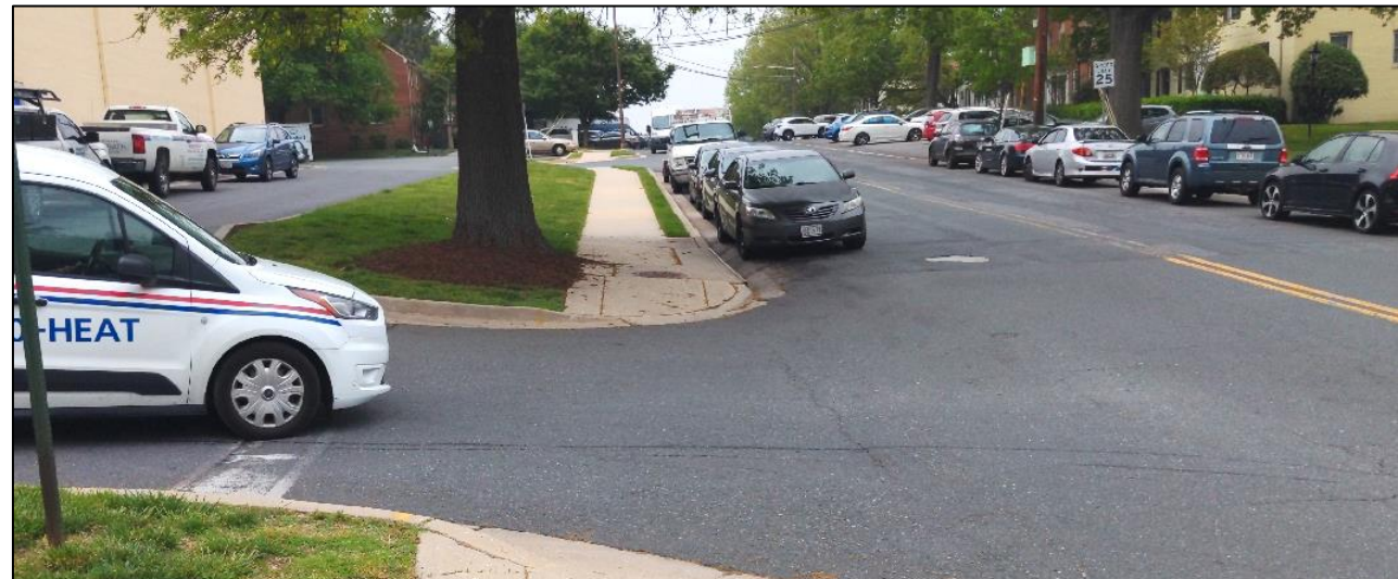
Washington Ave driveway with sight line limitations due to on-street parking (RCFES walkshed).
