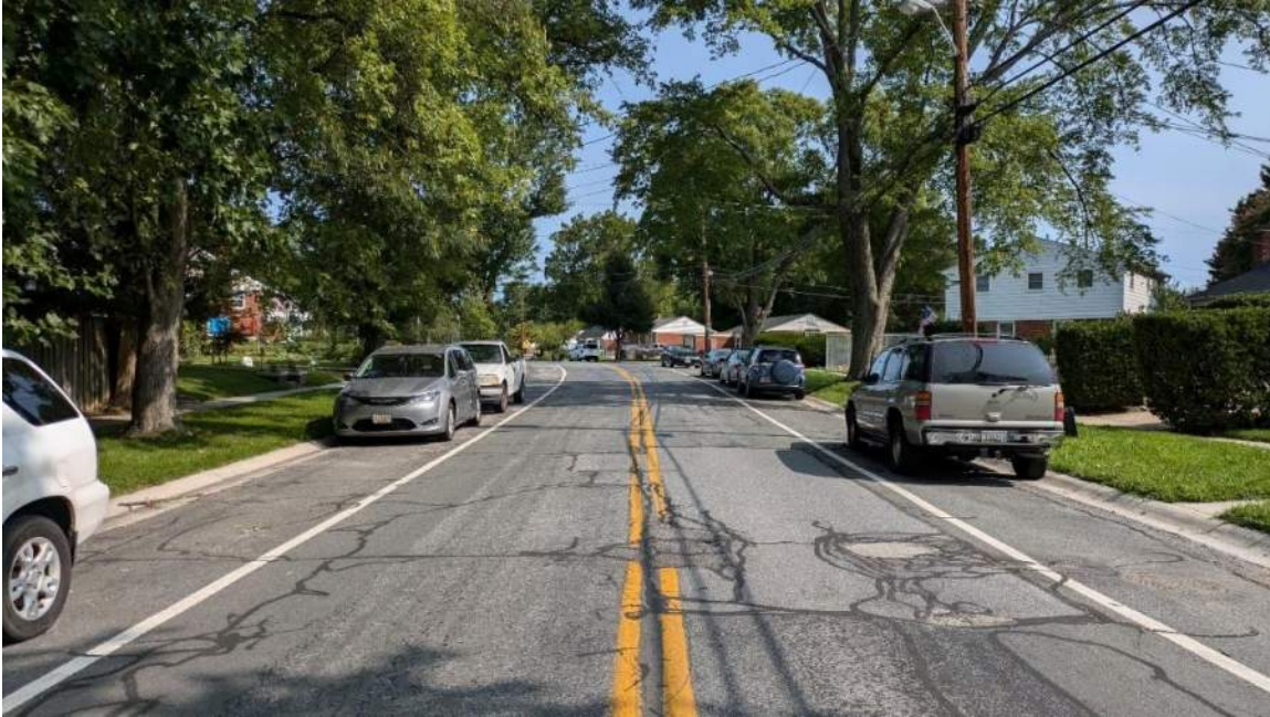
Photo 1. Bushey Drive looking north towards Elby Street. Approximate crash location.
