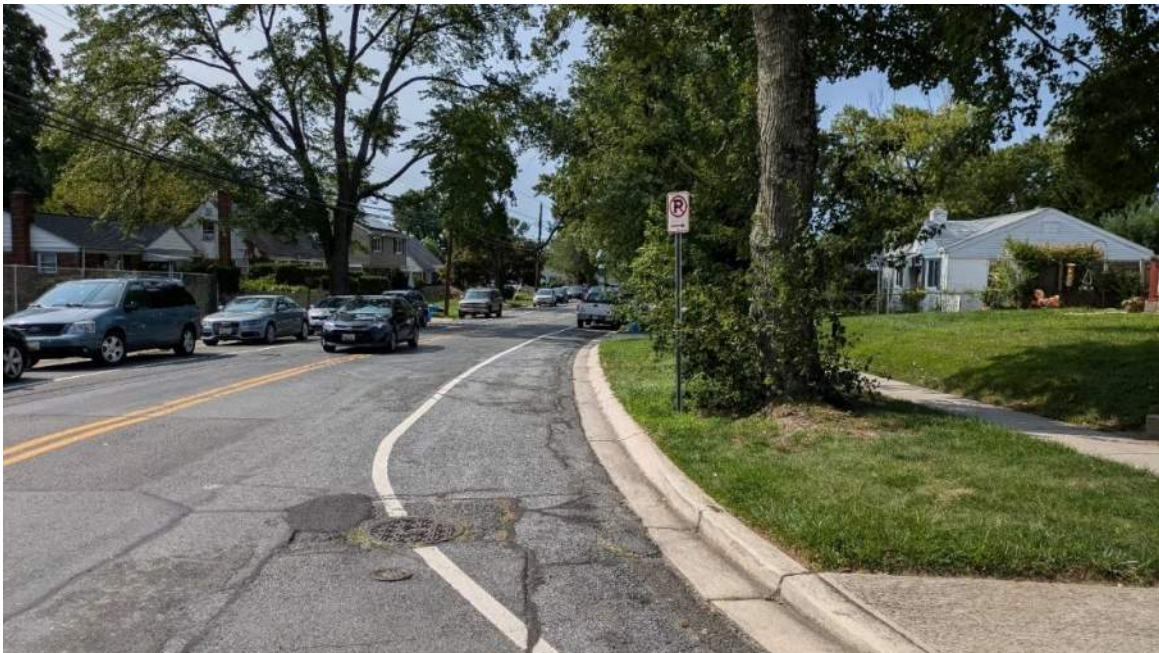
Photo 2. Limited sightline due to on-street parking and horizontal curve looking south along Bushey Drive from Elby Street intersection.
