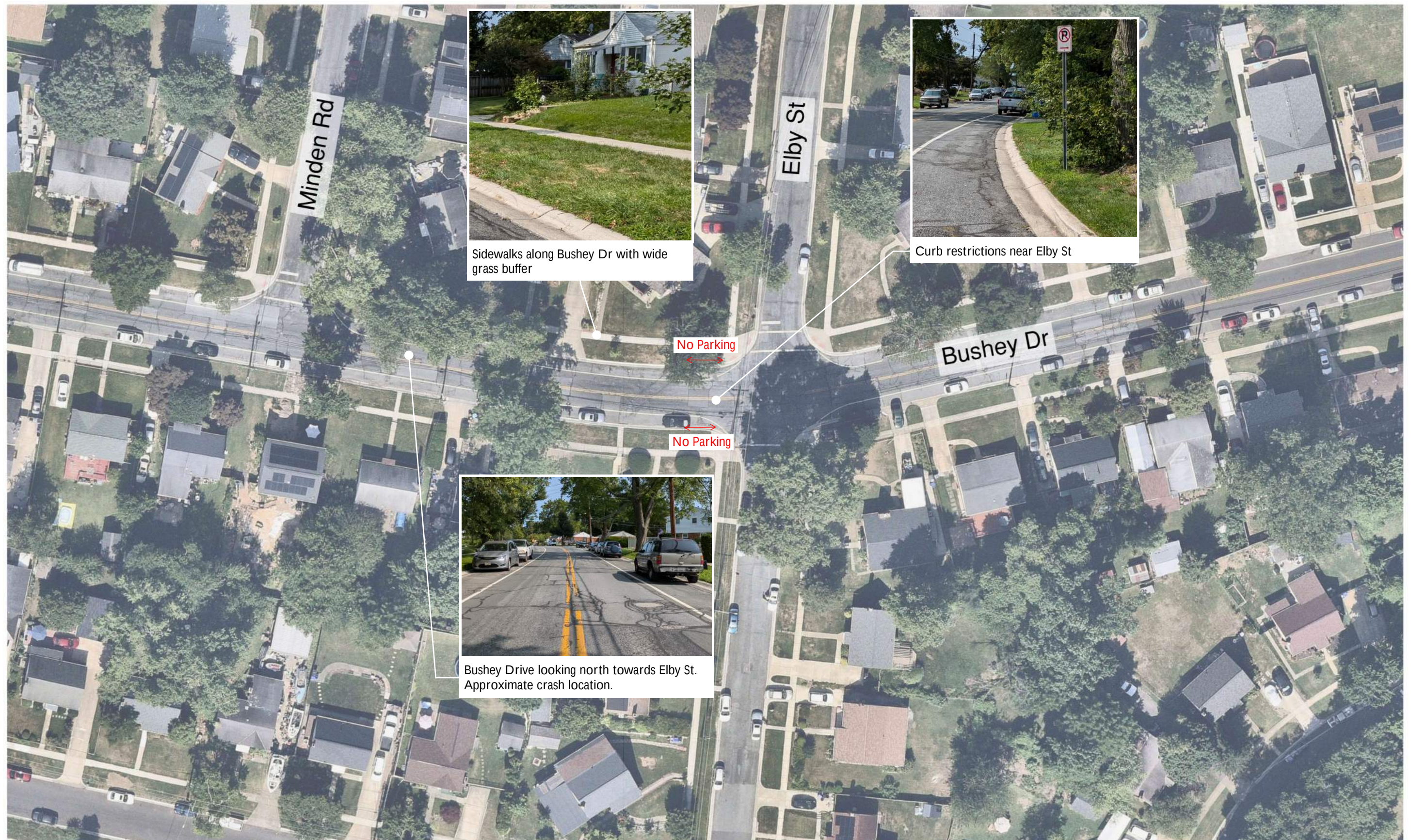
Figure 1 - Bushey Drive Corridor Observations
