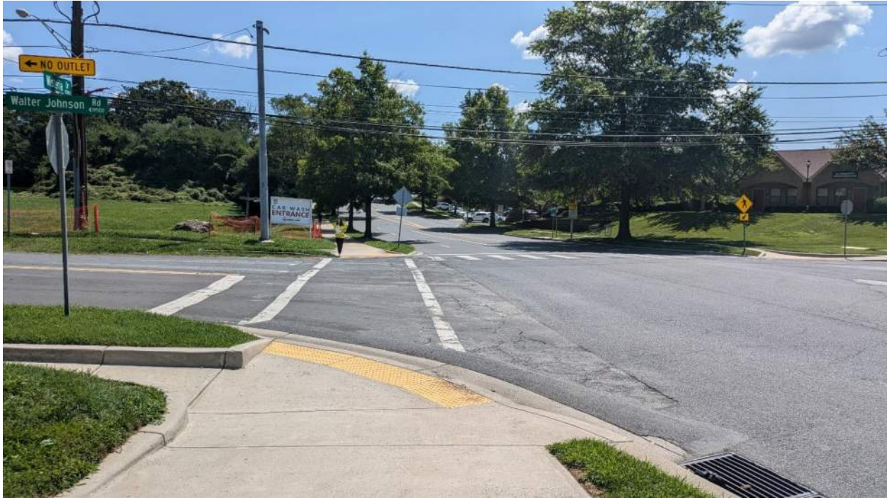
Photo 1. North leg of intersection where crash occurred, looking south along Wisteria Drive.
