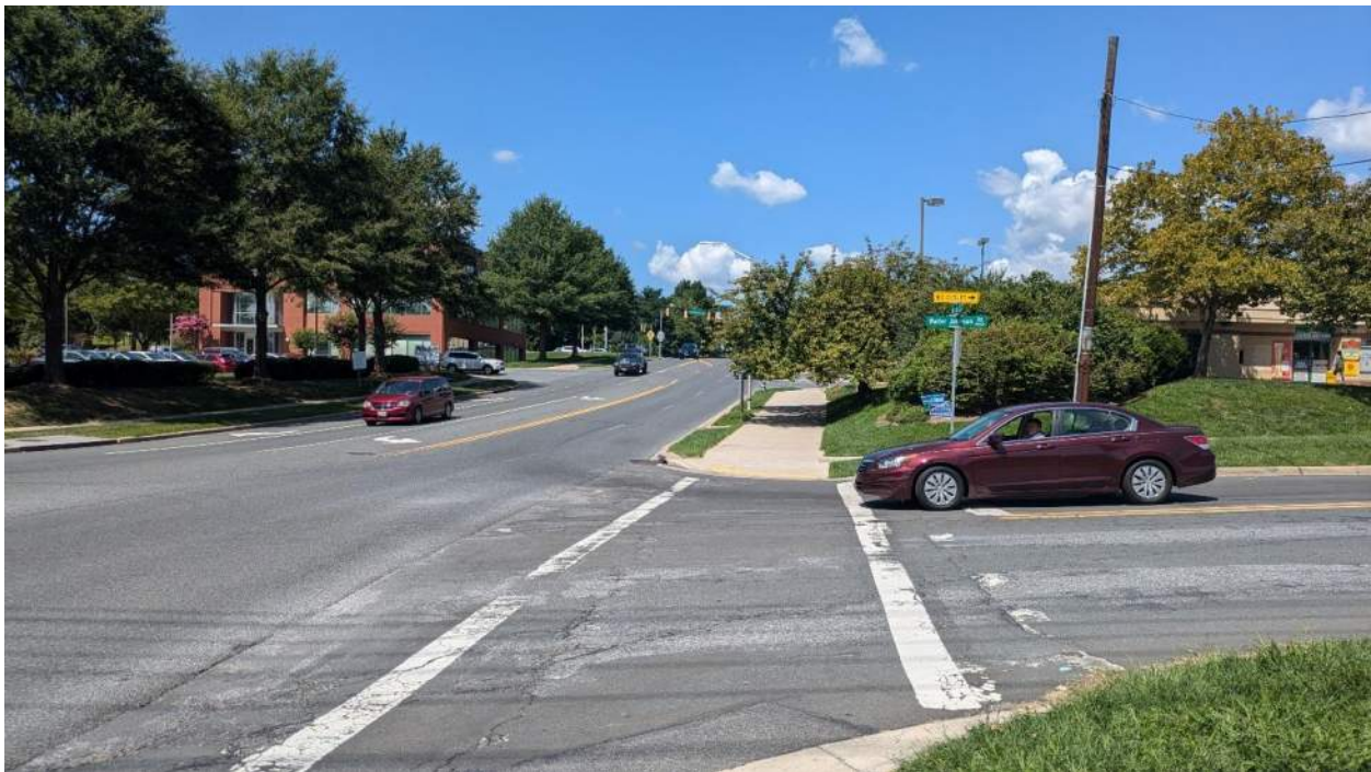
Photo 2. North leg of intersection where crash occurred, looking north along Wisteria Drive. Motorist can be seen creeping up past stop line before turning due to poor visibility.
