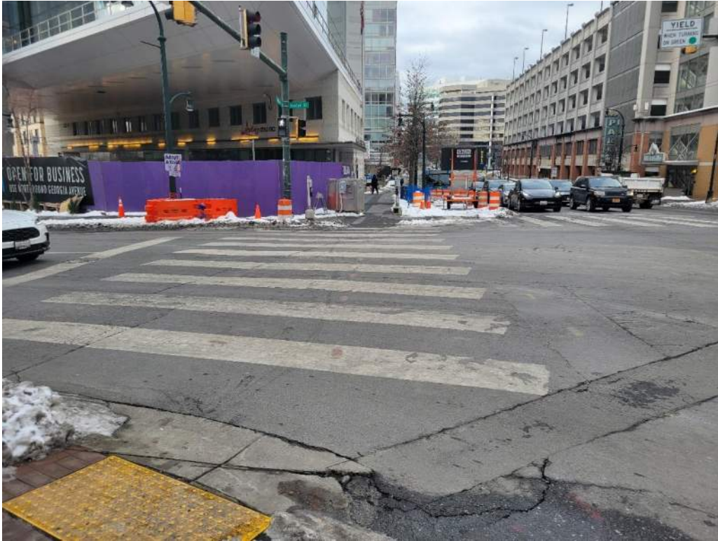
Photo 1. Taken from southeast corner looking westbound along Wayne Avenue at south leg crossing. Approximate crash location.
