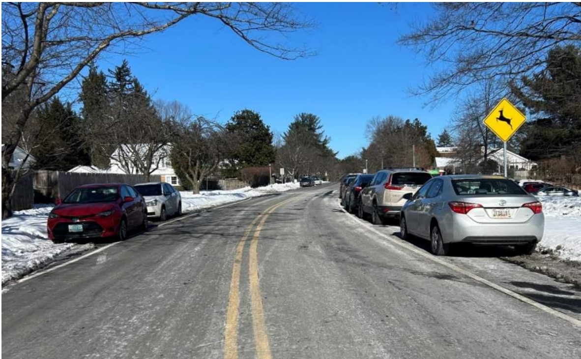
Photo 2. Limited sightline due to crest vertical curve looking north along Rippling Brook Drive towards Blair Stone Lane.
