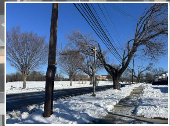
School flasher missing sign along Weller Road EB.
