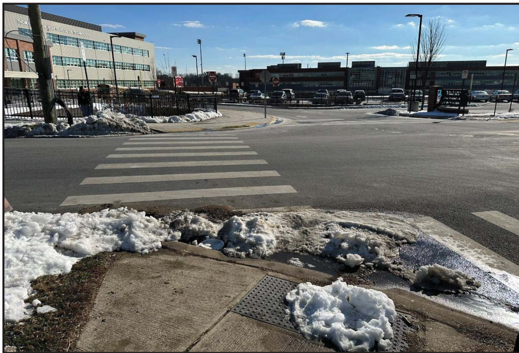
Photo 1. Crosswalk Markings at Dean Road Crossing
