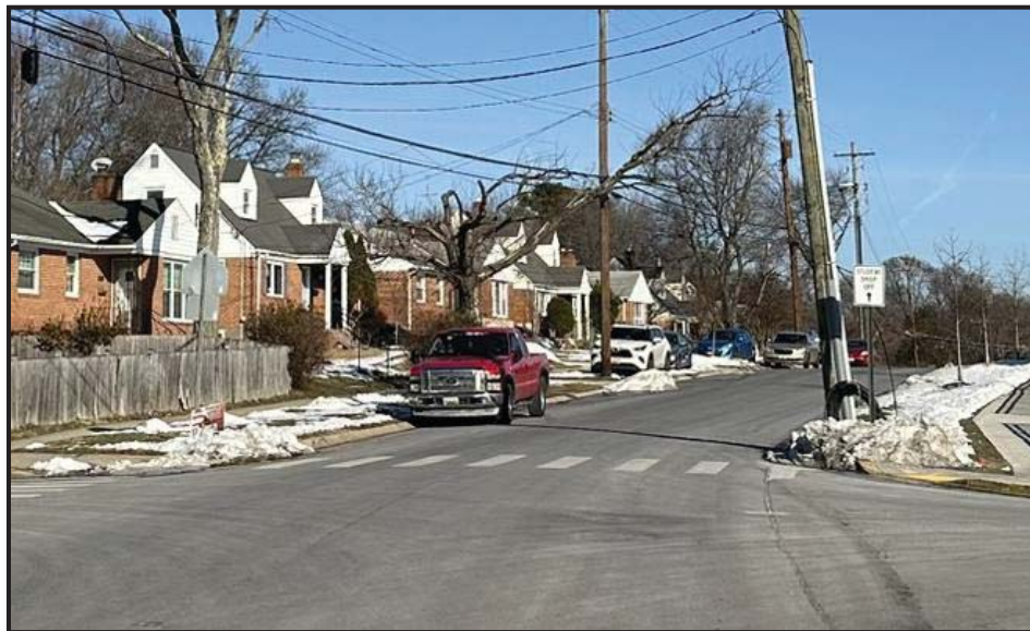
Photo 5. Absence of School Crossing Assembly on Eastbound Approach
