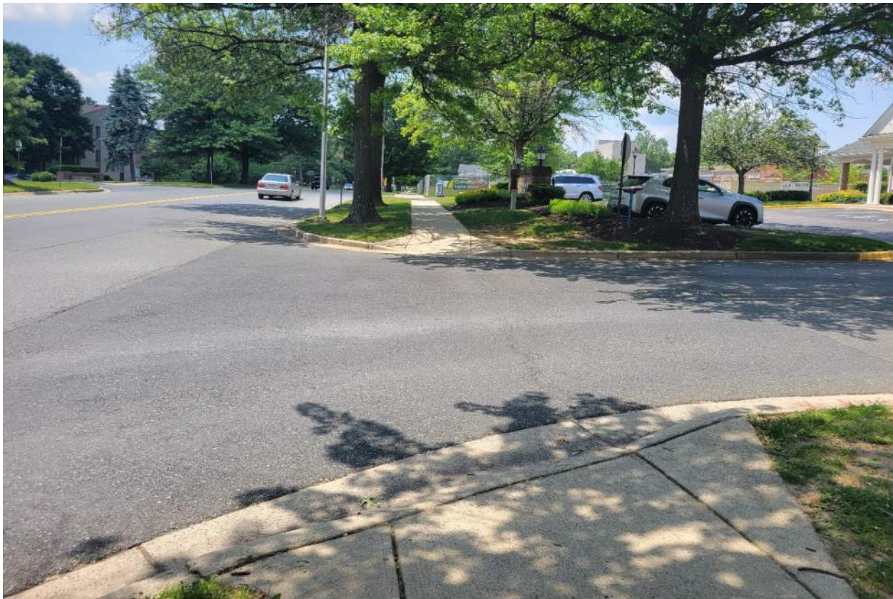
Photo 1. Taken from northeast corner looking westbound along Stedwick Rd. No pavement markings or detectable warning surfaces on ramps
