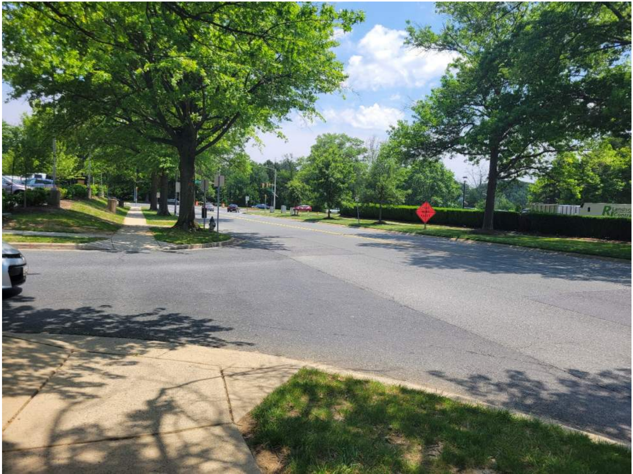
Photo 2. Taken from northwest corner looking eastbound along Stedwick Rd. No pavement markings or detectable warning surfaces on ramps.
