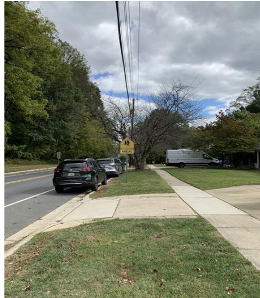
Figure 2: Faded school crossings and school ahead signs recommended for replacement
