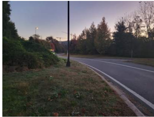
Bush slightly obstructs line of sight for pedestrians looking at off-ramp from the west
