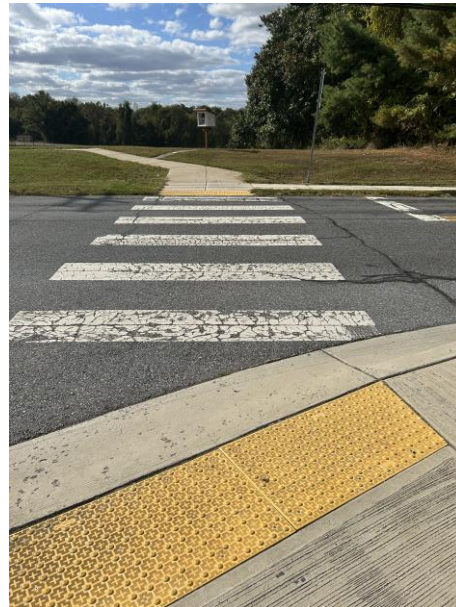
Figure 4: Photo taken looking west at northeast corner of Jones Lane / Falconbridge Drive intersection.
