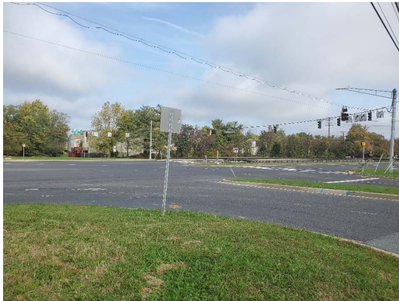
Picture 2: Looking across the west leg, showing the three-section and five-section signal heads for the Industrial Parkway approach and the two three-section ball and two three-section arrow signal heads for the northbound Columbia Pike approach.
