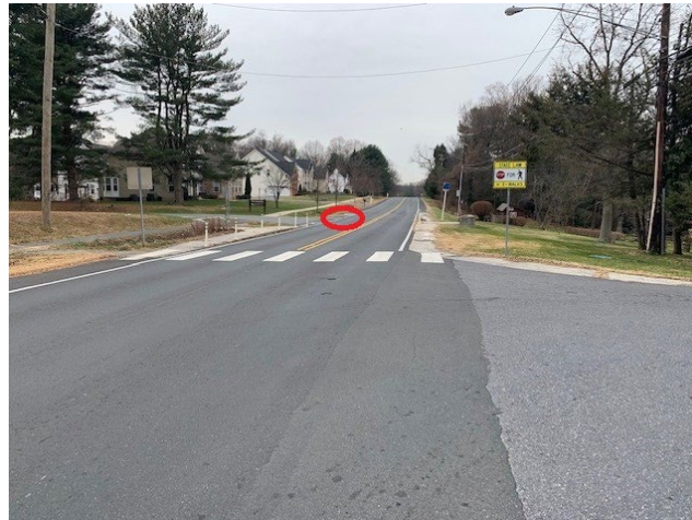
Eastbound Fairland Road near crash site
