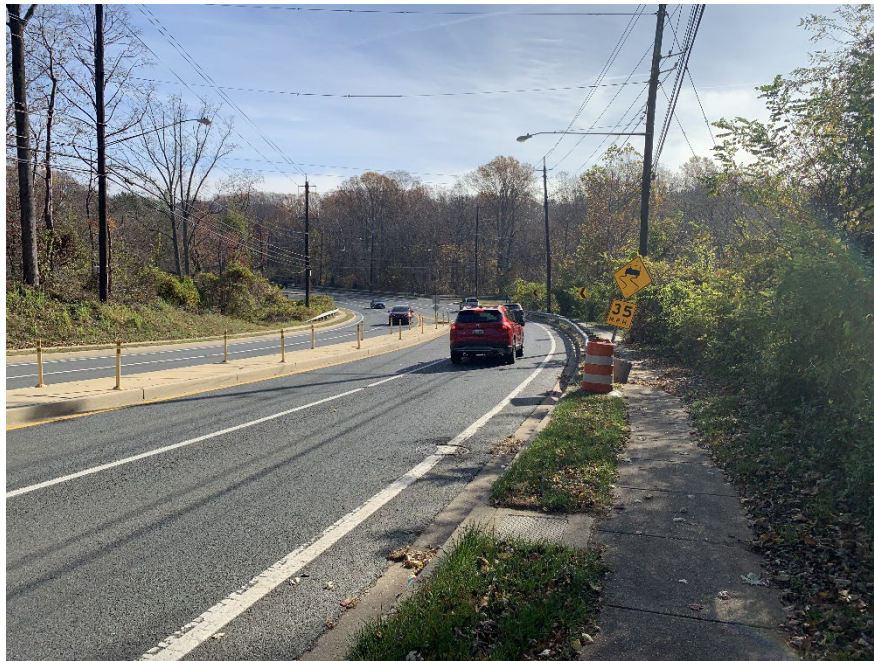
East Randolph Road at the Crash site
