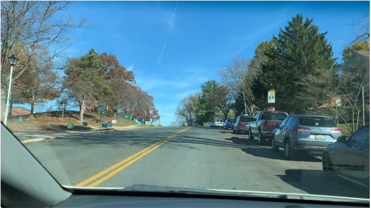
Eastbound School Drive, approaching flasher (approximately 450' west of crosswalk)
