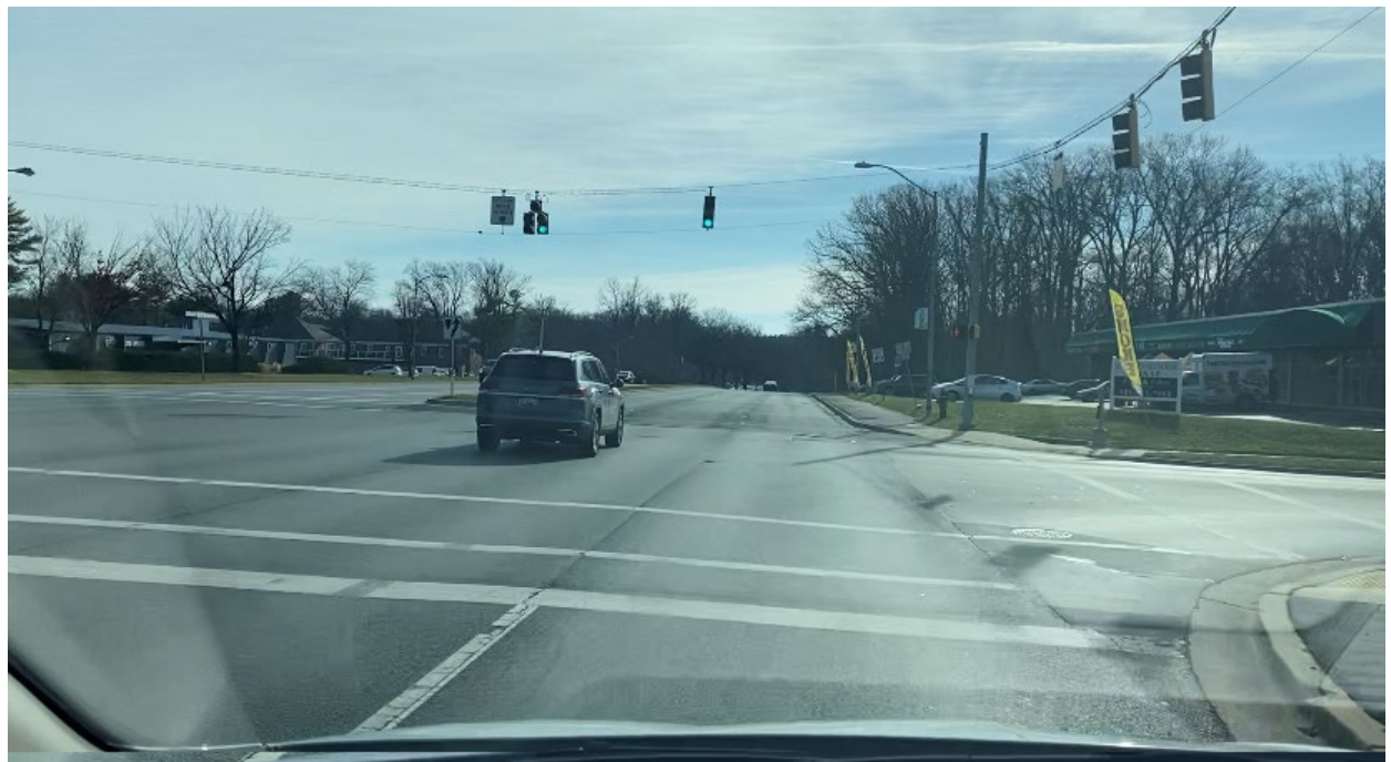
Eastbound East Gude Drive, at Taft Street
