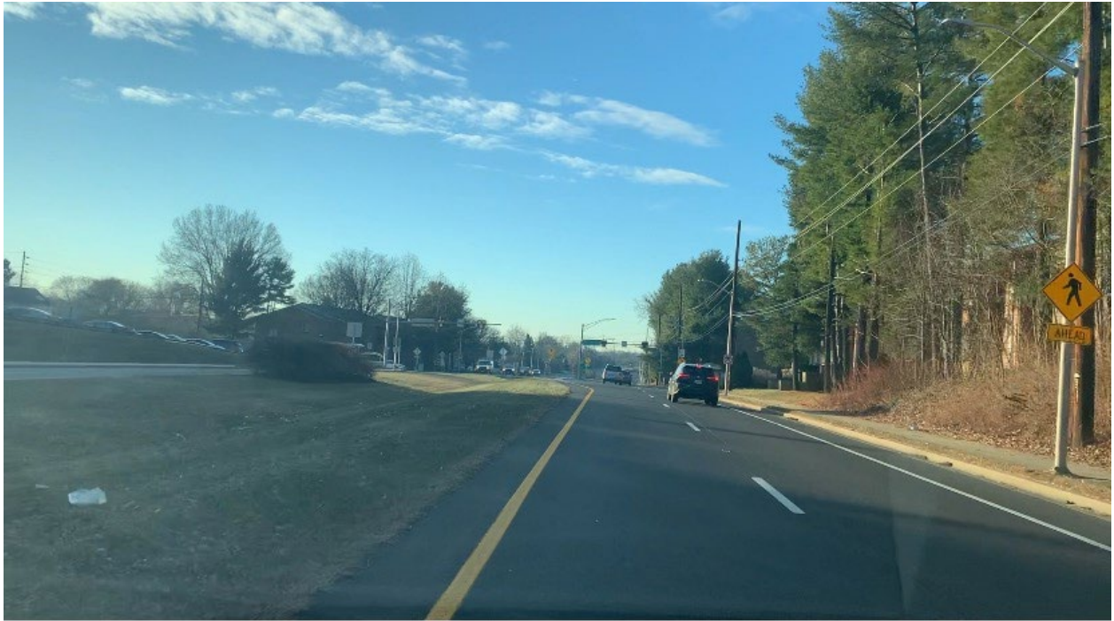
Northbound Muddy Branch Road, approaching King James Way
