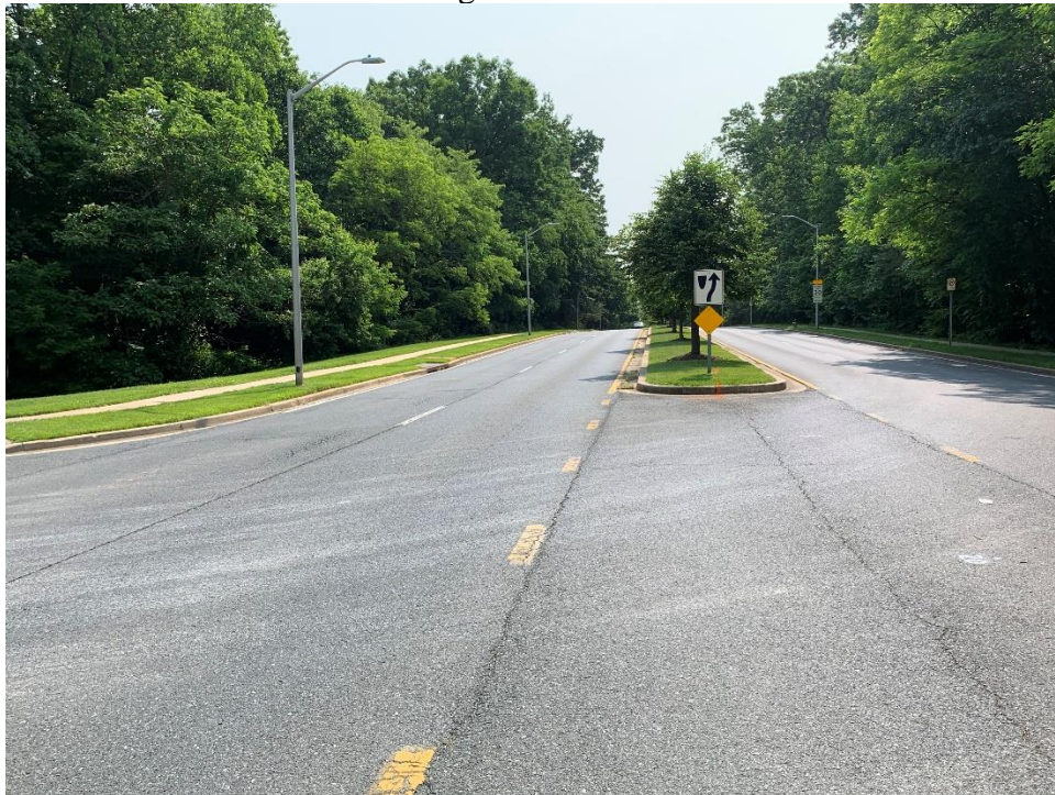
Eastbound East Village Avenue at Plum Creek Drive
