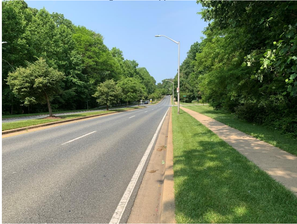
Westbound East Village Avenue approaching Plum Creek Drive
