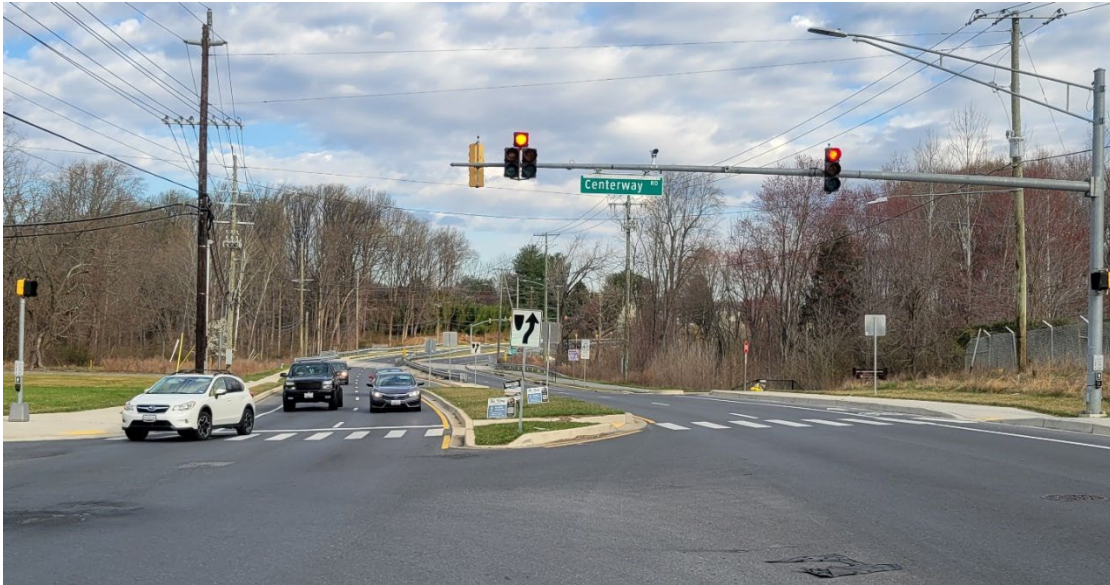
Northbound Snouffer School Road at Centerway Road
