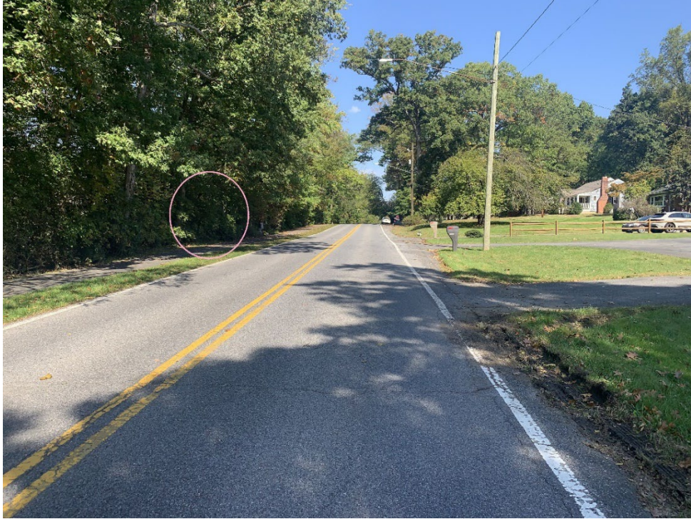
Northbound Norwood Road south of crash location
