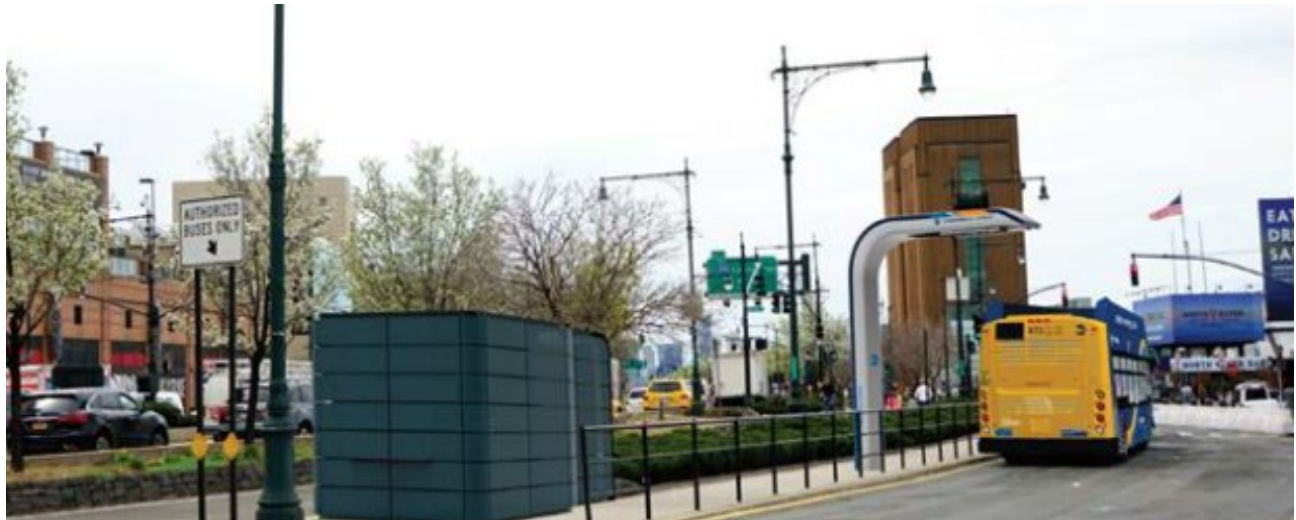
Figure 24: New York City Pantograph Charger
