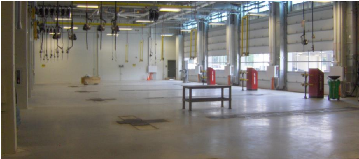
Figure 35: EMTOC Repair Bays with In-Ground Rotary Lifts
