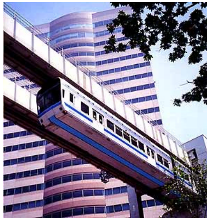
Figure 5.1. Suspended Monorail (Mitsubishi) Chiba City, Japan
