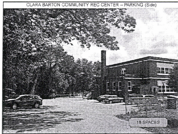
CLARA BARTON COMMUNITY REC CENTER – PARKING (Side)
