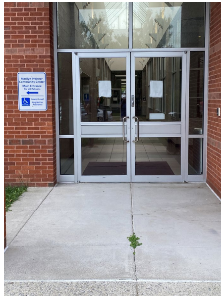
Right Side Entrance
