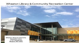
Wheaton Library & Community Recreation Center 11701 Georgia Ave Wheaton, MD 20902
