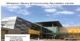
Wheaton Library & Community Recreation Center 11701 Georgia Ave Wheaton, MD 20902
