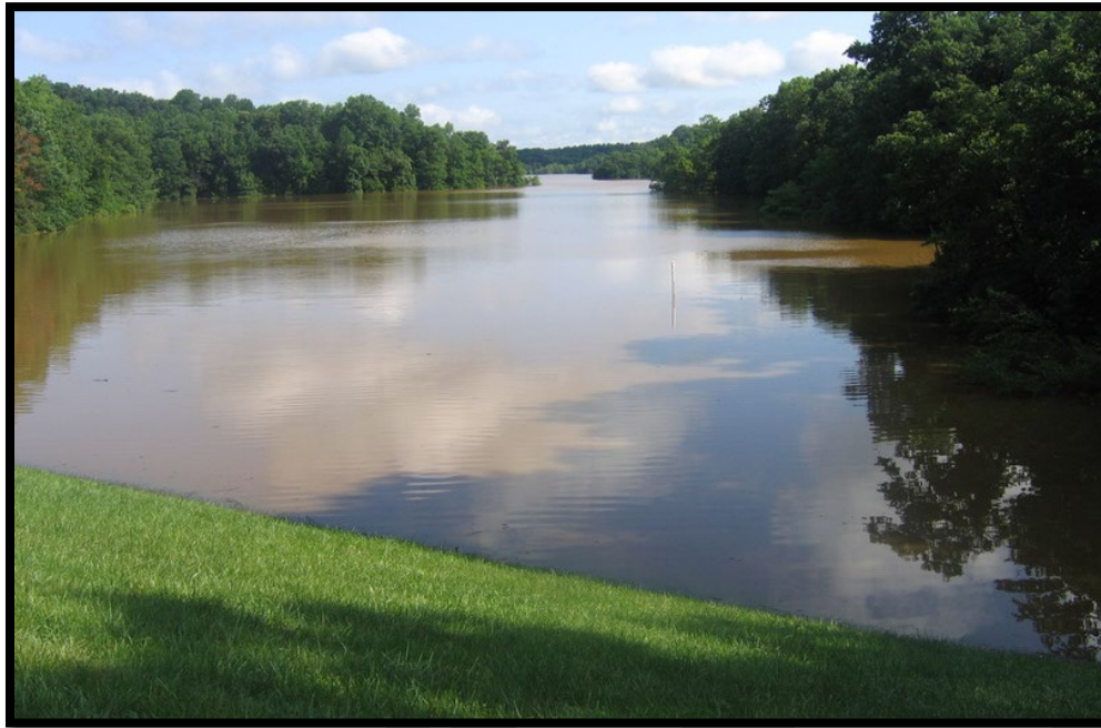
Figure 64: Lake Needwood Dam
