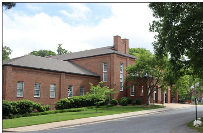
Figure 40: The Mondzac Performing Arts Center was built in 1989. It is located in the northwest section of the Landon School campus. EHT Tracerics.
