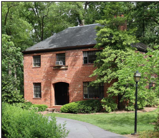
Figure 26: The Administration Building today houses the Admissions and Business Office. EHT Tracerics.
