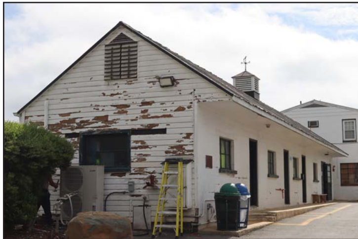
Figure 36: Foster Maintenance Building. EHT Tracerics.
