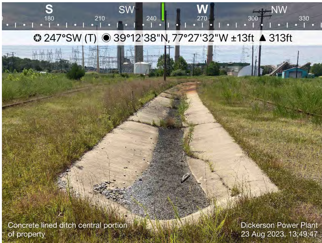
22. View of typical concrete-lined ditch in the central portion of the site (08/23/23).
