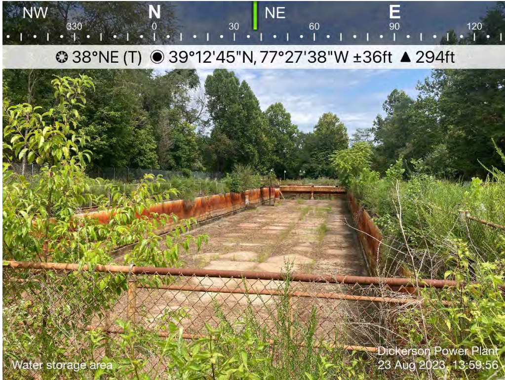
13. View of concrete-lined stormwater management basin (08/23/23).
