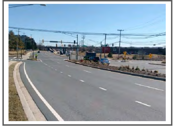
Intersection view along Sandy Spring Road facing west
