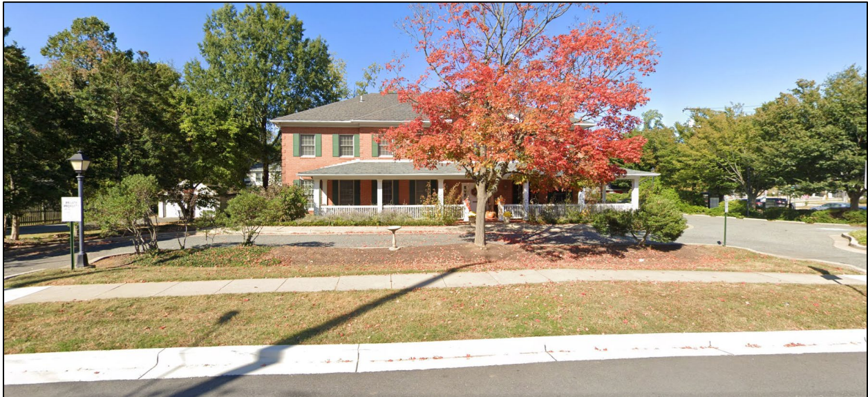
Figure 1: Subject Property viewed from Southwick Street
