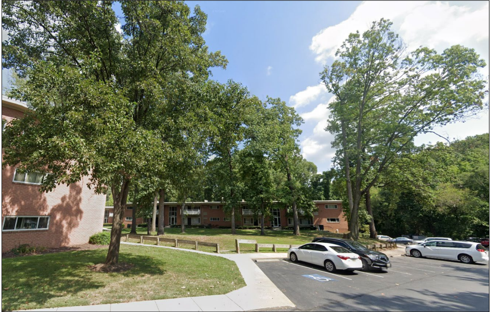
Figure 4: Glenmont Forest Apartments Existing Conditions
