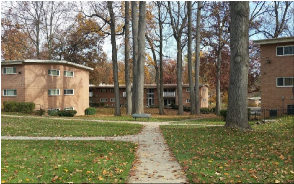
Figure 5: Glenmont Forest Apartments Existing Conditions
