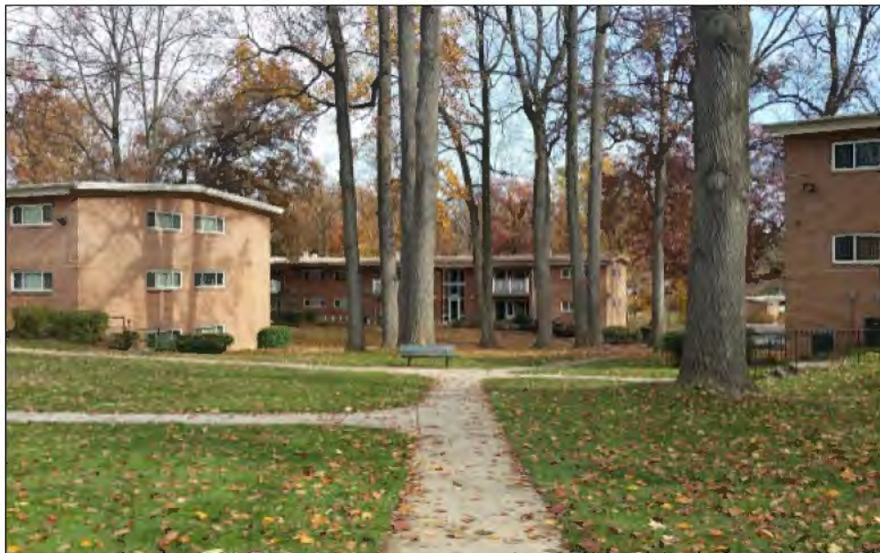
Figure 5: Glenmont Forest Apartments Existing Conditions
