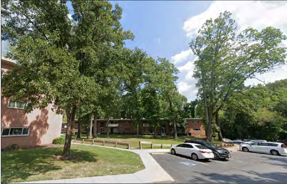
Figure 4: Glenmont Forest Apartments Existing Conditions
