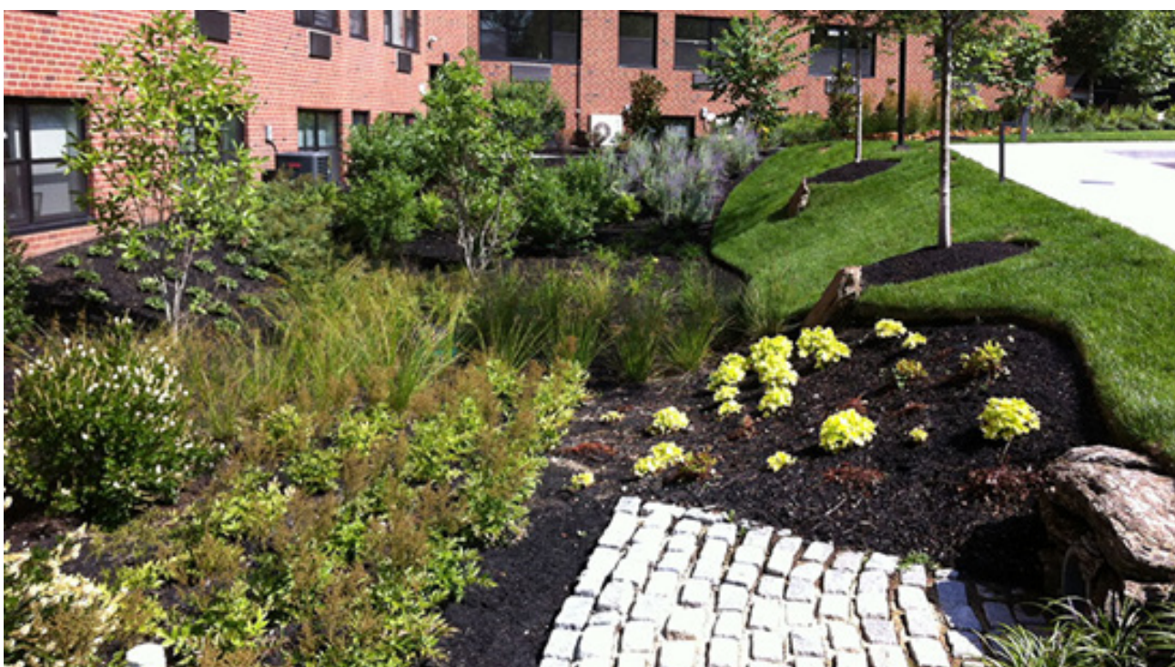
Figure 19: Micro-Bioretention Planting
