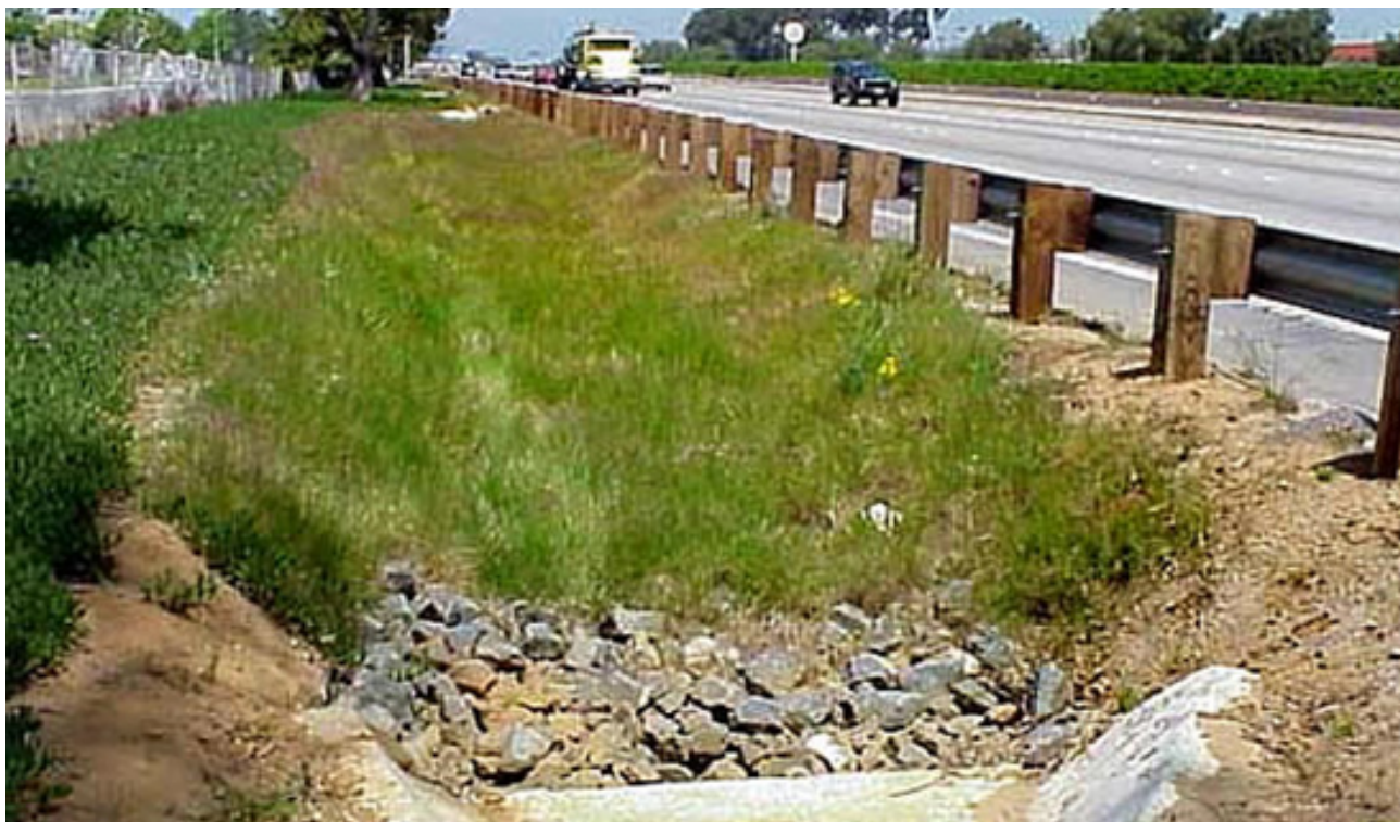
Figure 18: Biofiltration Swale
