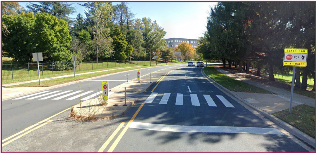
Figure 7: View of pedestrian crosswalk at Crabbs Branch Way
