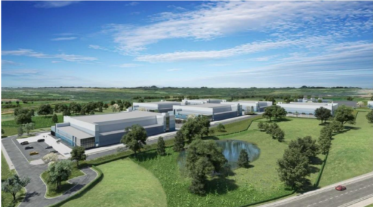
Exhibit 16, pg. 2 “Exhibit 7” – Data Center
