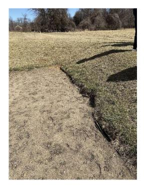
Repair all failing interior slopes and provide clean grading transitions to the filter media.
