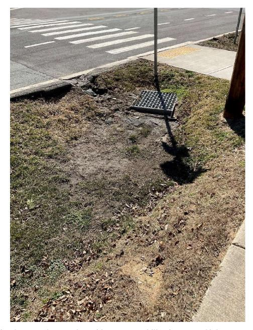
Repair erosion from roadway and provide proper stabilization around inlet.
