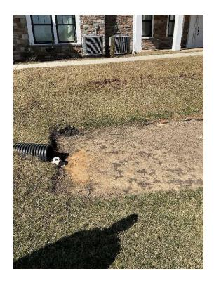
Repair all failing interior slopes and provide clean grading transitions to the filter media
