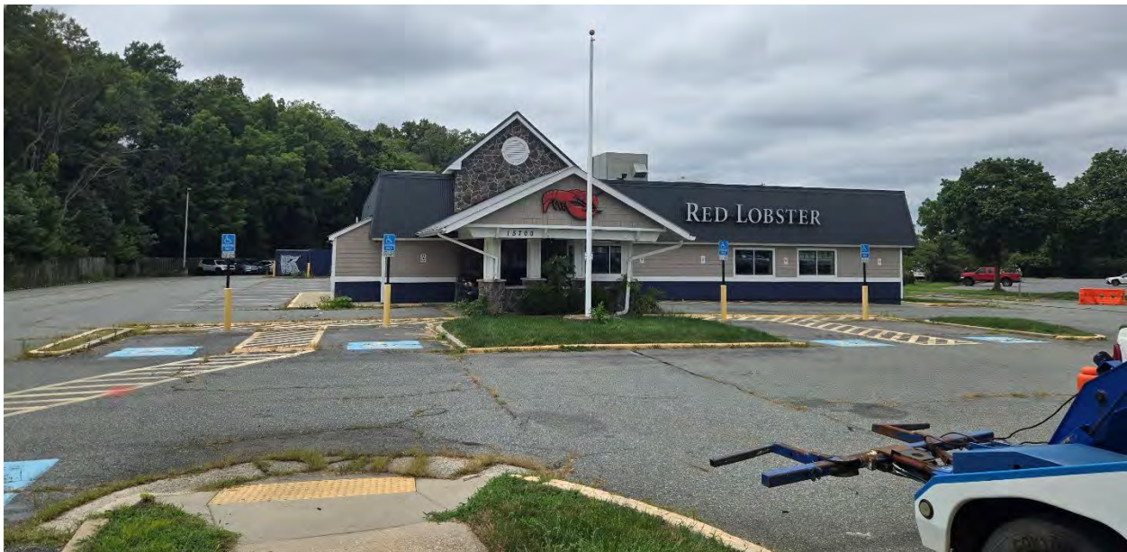
Former Restaurant from access road (Shady Grove Rd to the left)
